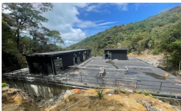
Figure 5. Wastewater treatment station of Ba Na tourist area
