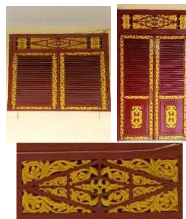
Figure 7: Wajik-Wajik Ornament Above the Door and Window as Ventilation
