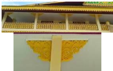
Figure 15: Elbow Ornament Located at the Top Corner of the Pole
